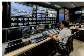
▲ Kairos Control panel used by Yomiuri Telecasting Co.
