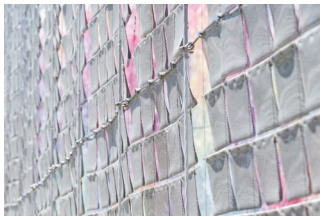
▲ The fabric panels are programmed to sway dramatically when visitors inside the pavilion smile
