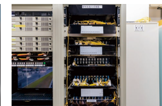
▲ Camera video feeds transmitted via optical fiber to East Control Room.
