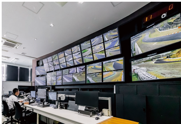
▲ In the East Control Room, camera feeds are monitored on ten screens, including six with multi-view displays.
